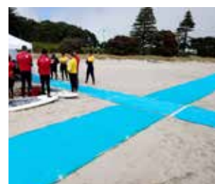
X-beam crossing with right angles
